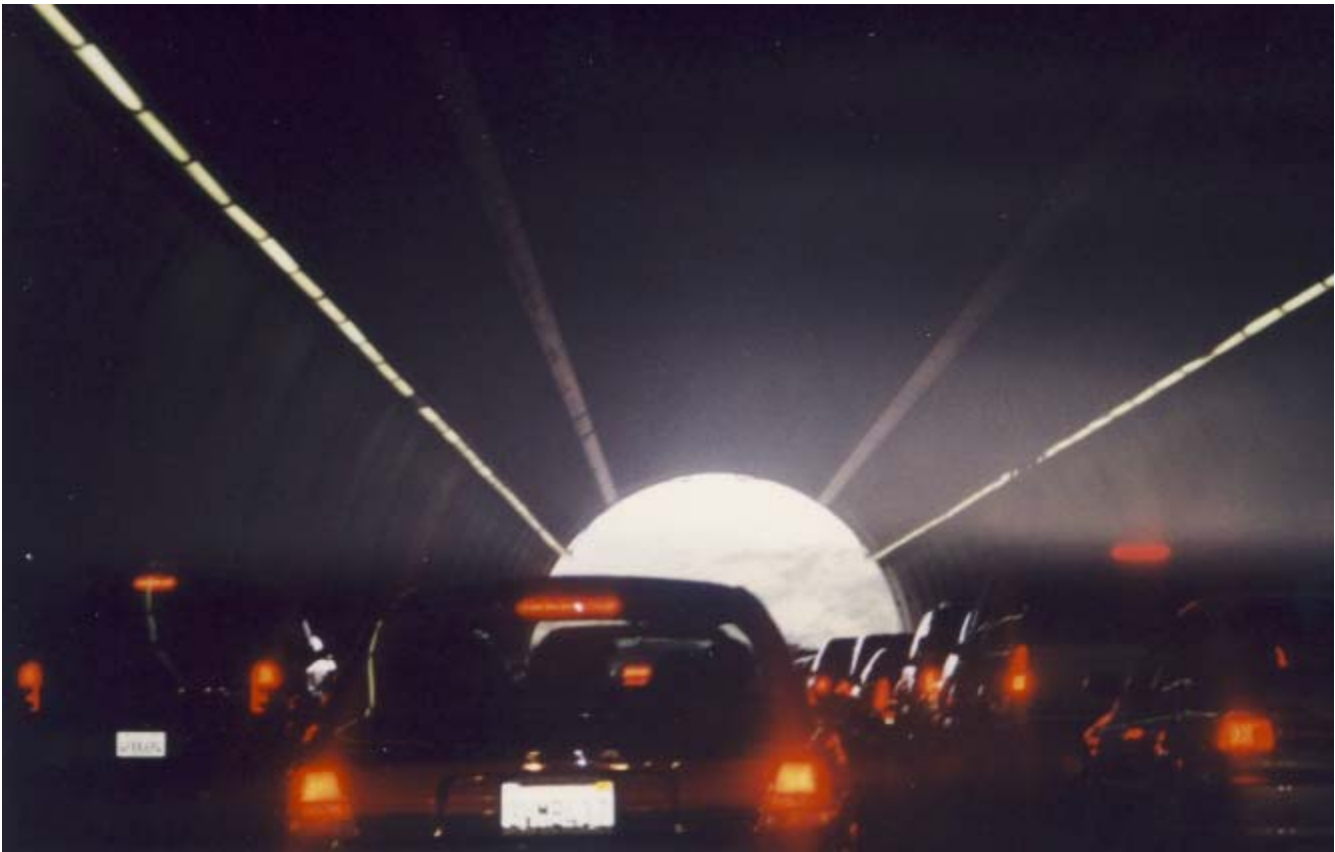
Roadway Tunnel, California
